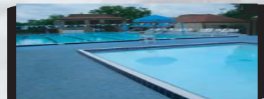
WESTMONTE PARK RECREATION CENTER SWIMMING POOL
